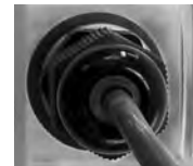
Cable Gland with cable
